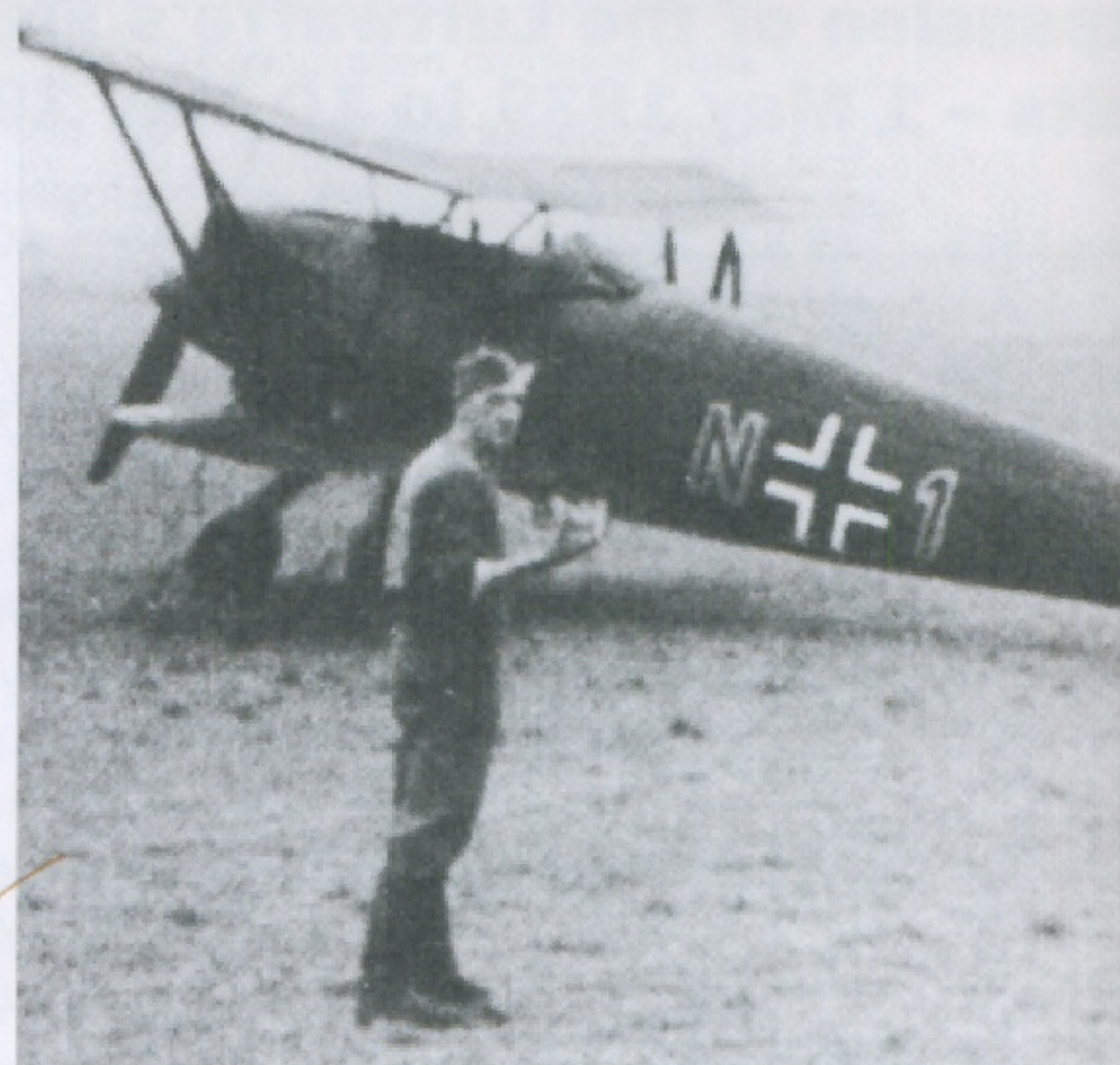
ABOVE: An Arado 68 F-1, probably seen at Oedheim/Heilbronn in September 1939. The machine was fitted with flame dampers for nocturnal operations.
